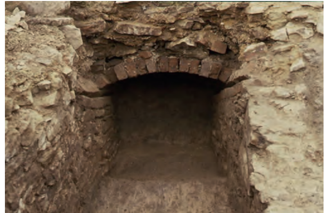
Fig. I/15: Chrudim, Filištínská St., cesspit XVIII. Drainage of sewage through the town wall with a brick arch. 16 th century.
